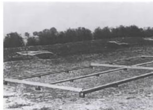
02 WOODEN BEARERS ARE LAID ON LEVEL GROUND
