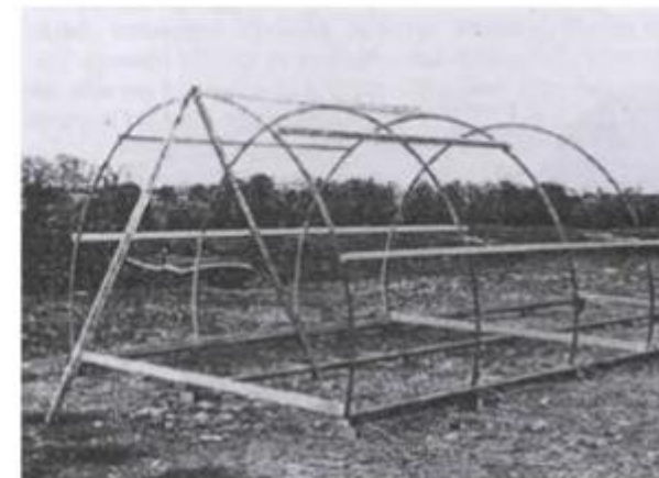
03 STEEL RIBS BOLTED TO BEARERS
