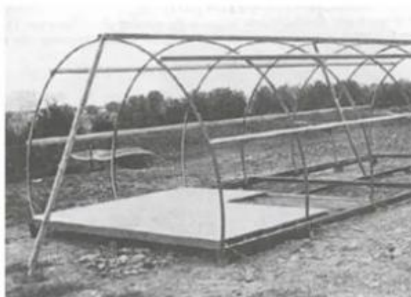
04 WOODEN JOISTS SCREWED TO BEARERS SUPPORT FLOOR
