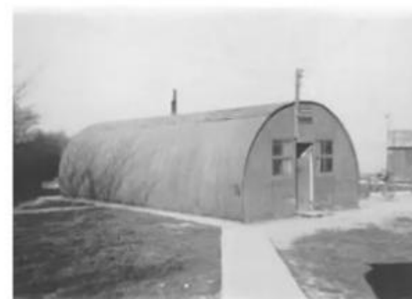
06 OUTER CORRUGATIONS FIXED AND ENDS COVERED
