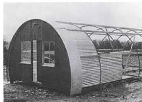
05 INNER LINING OF LIGHT CORRUGATIONS FIXED
